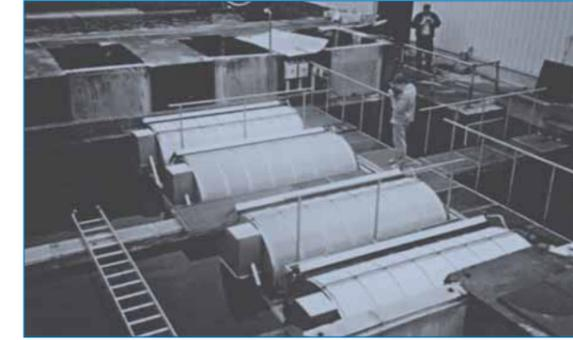
Hydrotech's patented filter elements greatly simplify both the replacement of the elements and the change of the filter opening size. The drum is constructed in sections, each with three, four or five filter elements depending on the diameter. This facilitates maintenance operations and makes it easy to adapt the filter to the actual need of flow capacity and performance requirements of filtration.
